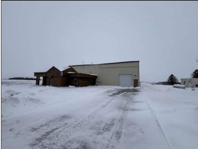
Photo 1 – View of the building looking west
